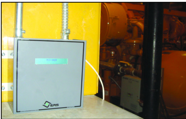
▲ The Monitoring & Control Server manages the collection and flow of data gathered from sensors in a building’s utilities infrastructure.
